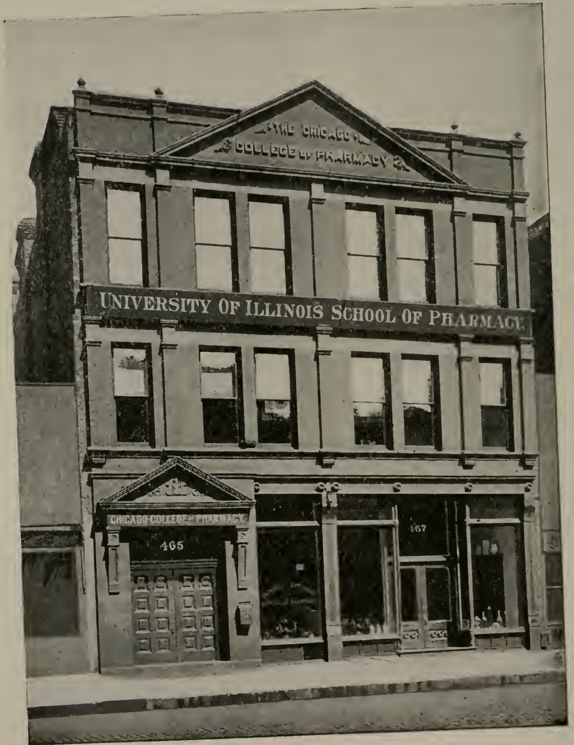
THE SCHOOL OF PHARMACY BUILDING
